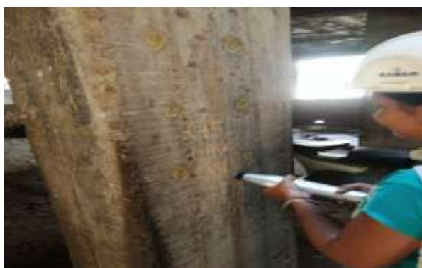
Fig. 2. Rebound Hammer Test
