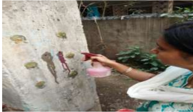
Fig. 4. Depth of Carbonation Test
